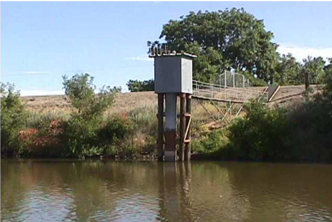
Figure 11: The DWR Brandt Bridge Station
