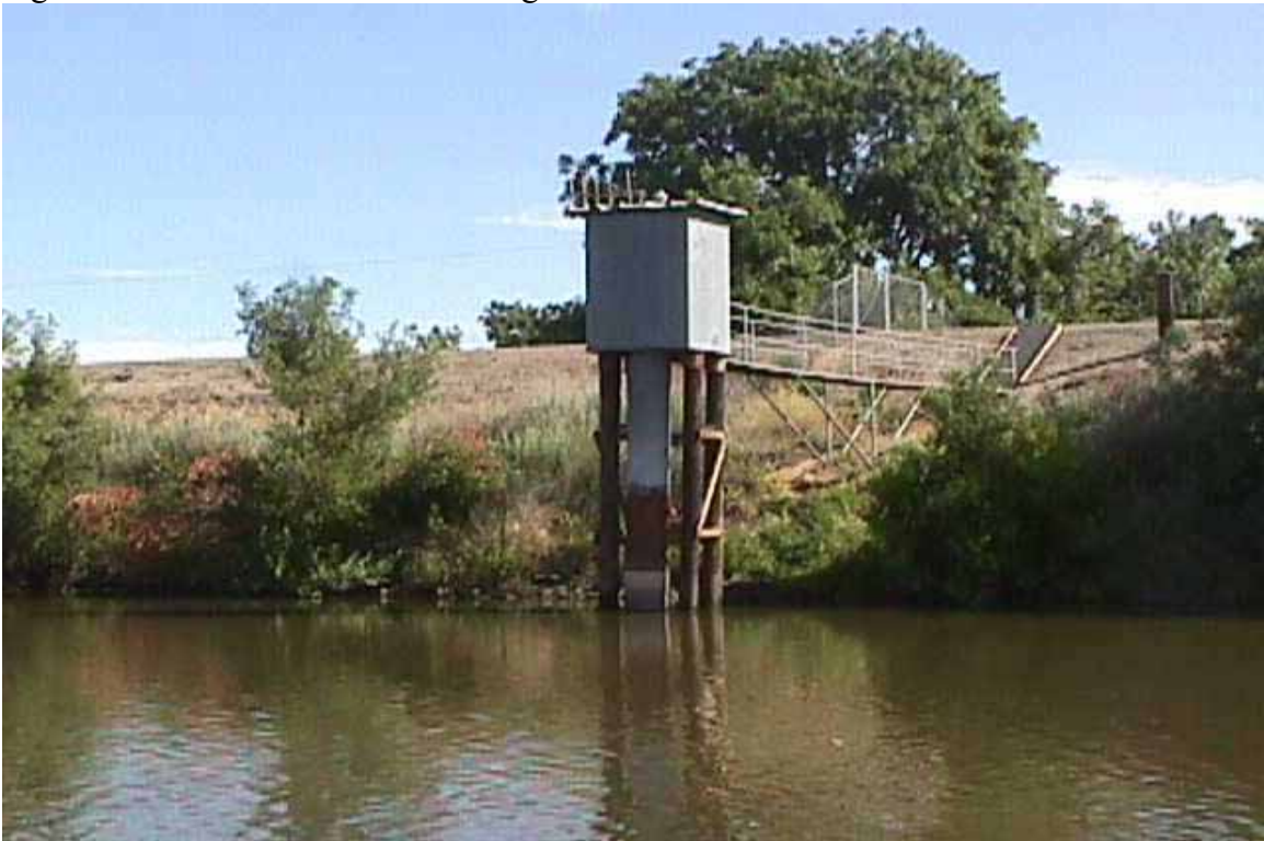
Figure A-14: Piers used at OP for chain-mounted sonde deployment.
