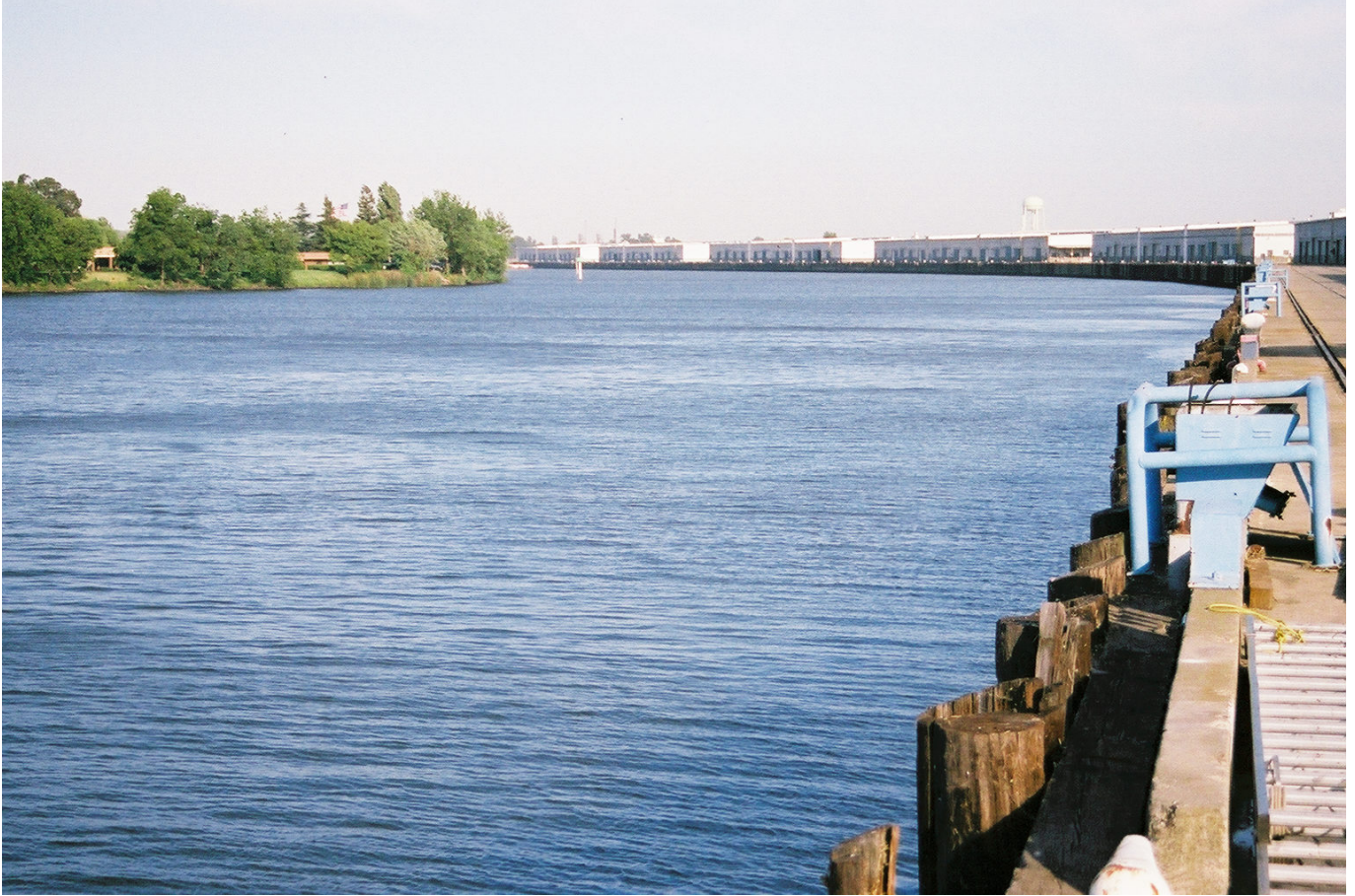
Photo 1: Upstream View of the Port of Stockton's Rough & Ready Island Dock.
