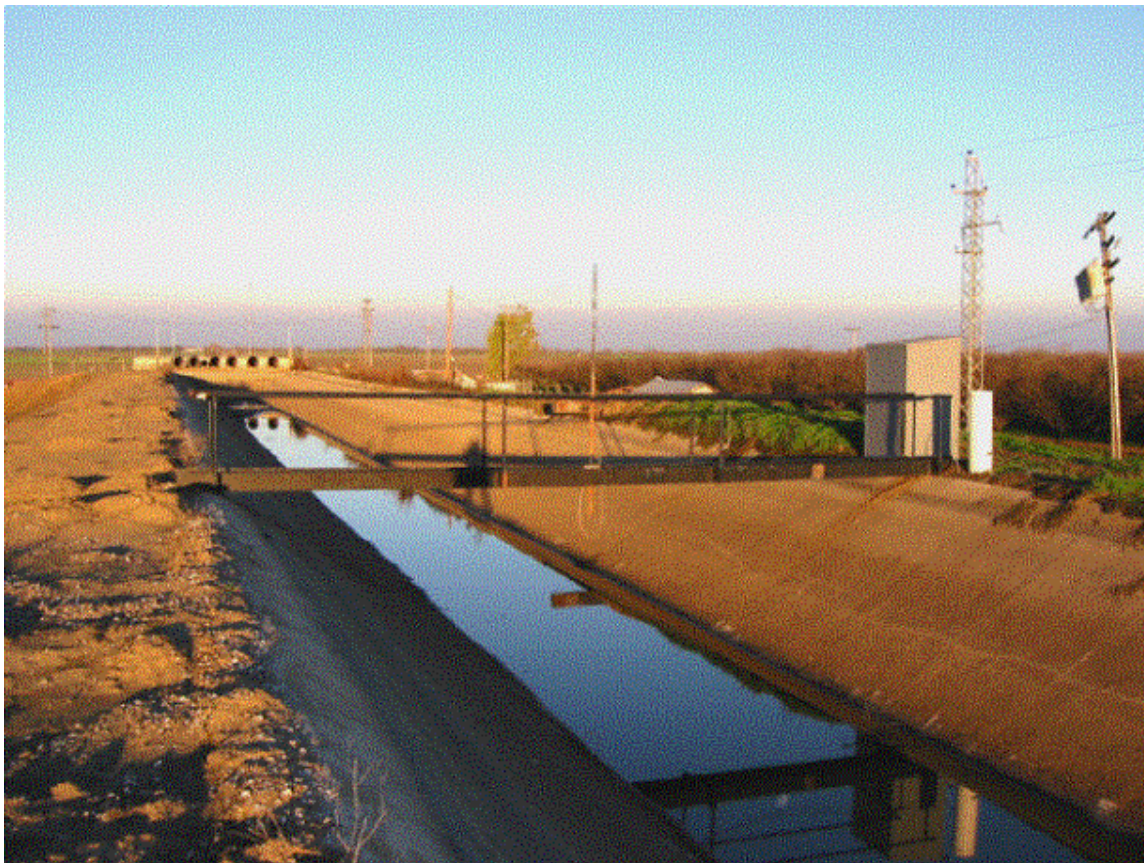
Figure I-1. Flow and water quality monitoring station at the West Stanislaus Irrigation District.
