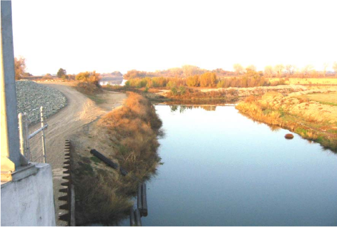
Figure J-1. Banta Carbona Irrigation District intake canal.
