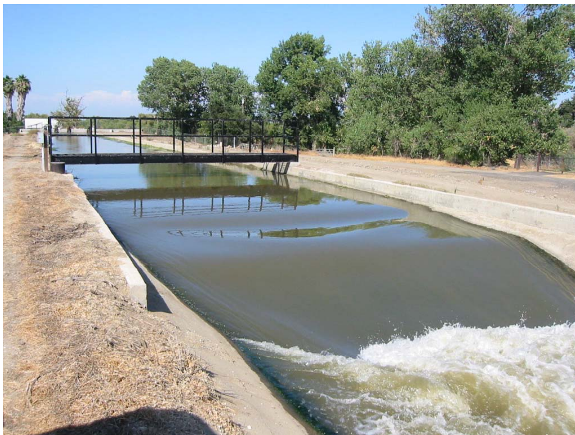
Figure I-2. Flow measuring flume at the Patterson Irrigation District.
