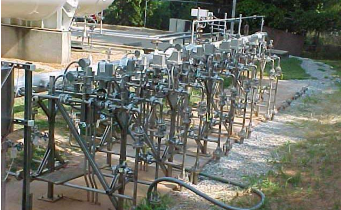
Richard B Russell Oxygen Distribution and Flow Control Manifold
